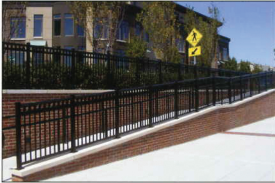
Traditional Style Railing with ring design and ADA Compliant Handrail, community park
