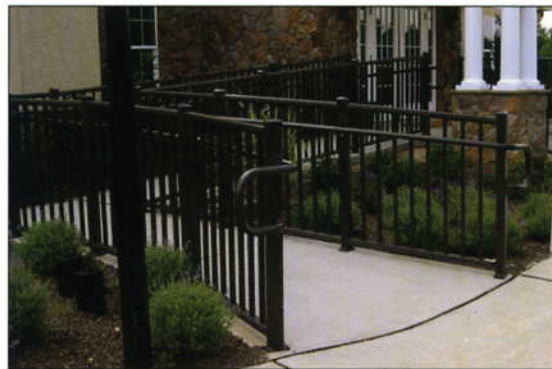
Colonial Style ADA Compliant Ramp Railing, community center
