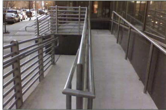
Custom ADA Compliant Ramp Railing, high-rise residential
