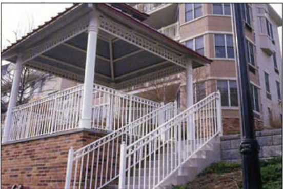
Traditional Style Railing with rings at waterfront entrance, luxury multi-family residences - Jersey City, NJ
