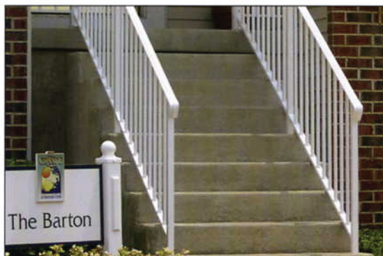
Standard Style Railing at front entrance, new single-family community - Rancocas, NJ
